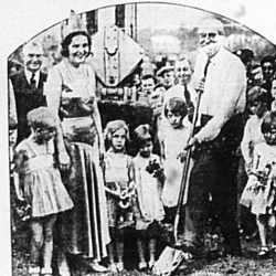
Gov. Wallace H. Hoge, accompanied by other officials, breaks ground for the new Pinchot dam on the St. Lawrence river. The dam will be 300 feet long and 17 feet high. It is the largest dam ever built in the state.
