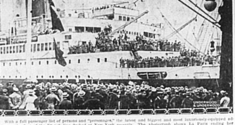
View of a full passenger list of the new liner...
